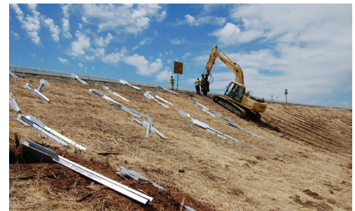
Williams, California: Stabilizing 1.5 miles of ramp slopes for CA DOT
