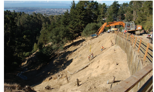
Oakland, California: Steep slope stabilization
