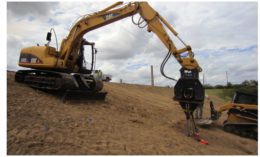
New Madrid, Missouri: Levee repair
