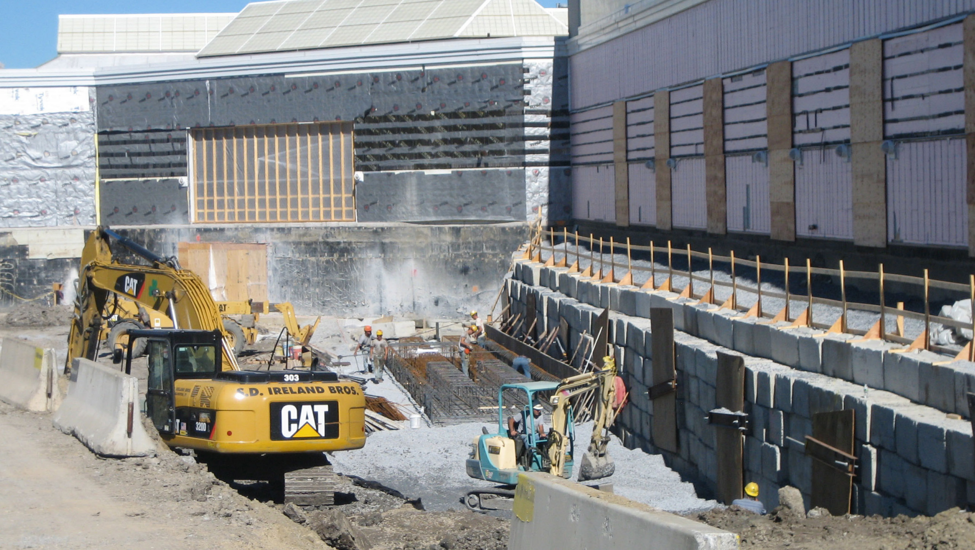
East side footing construction is underway next to concrete block retaining wall built to protect ice hockey arena footings.
