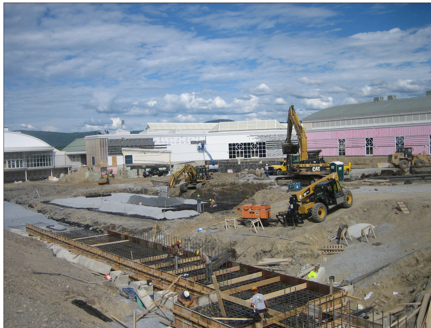
Workers in foreground build concrete forms for west side footings while mass excavation and placement of aggregate base for building slab take place in background.
