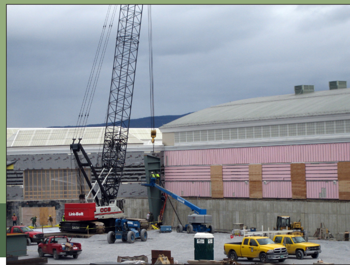
CCS Constructors uses a Link Belt crane to erect first 36-foot-tall steel column on east side.
