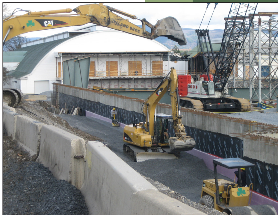
S.D. Ireland Company backfills foundation wall as part of its subcontract to perform all site work at the new facility.
