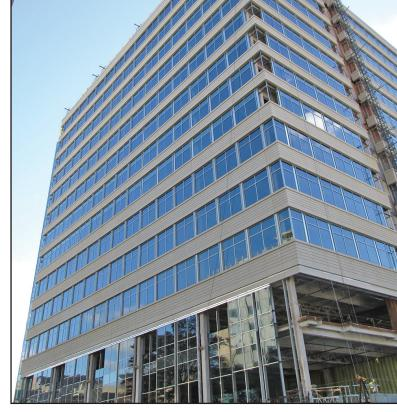
delivering them as needed each night while the steel frame was erected during the day. The panels were staged at a temporary storage facility near the actual site, which was too constricted to allow panels to be delivered there. The panels were picked from the trucks as they arrived and hoisted into place immediately by the tower crane. Coreslab Structures (CONN) Inc. in Thomaston, Conn., fabricated
