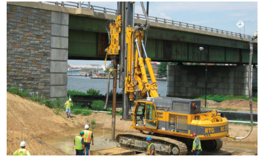
11th Street Bridge Washington, D.C.
