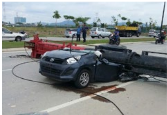
► Accident Involving a Piling Rig Image source: Guide to Working Platforms By the Joint EFFC/DFI Working Platform Task Group 1st Edition December 2019
