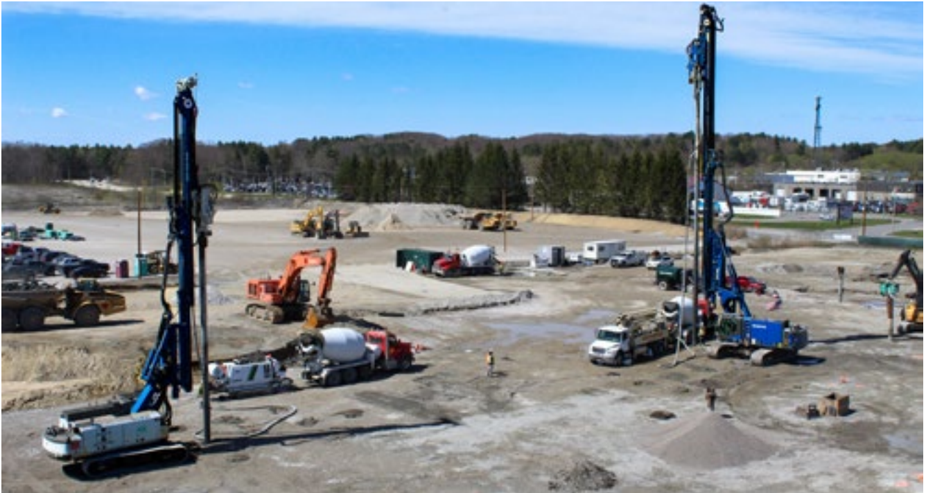
▶ Two Geopier® GeoConcrete® Column (GCC) rigid inclusion crews operate on a well-prepared Working Platform.
