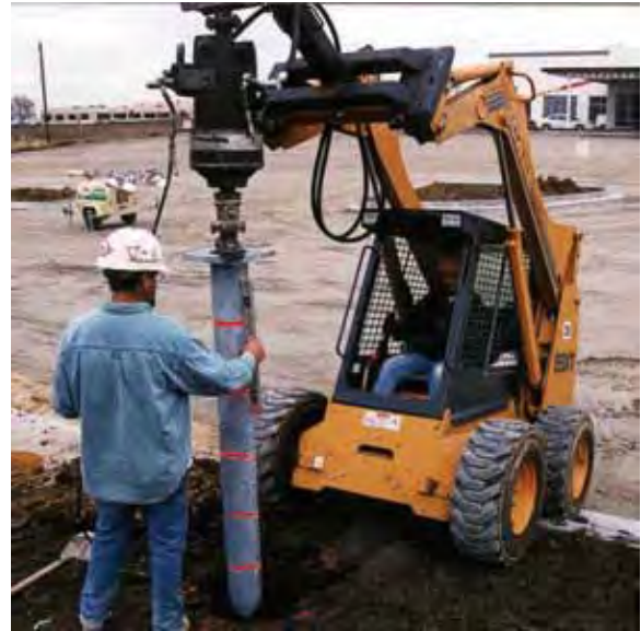
Foundation Lighting and Signs® Products are Easily Installed Using Common Construction Equipment. Figure 10-3
