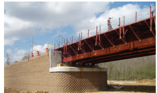
I-10 and Picardy Avenue Interchange Baton Rouge, Louisiana
