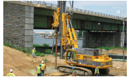
11th Street Bridge Washington, D.C.
