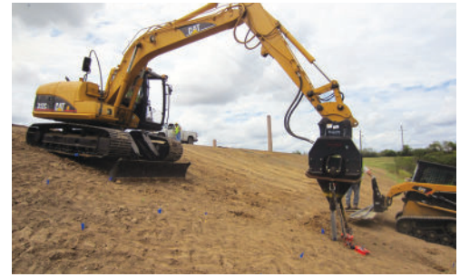
New Madrid, Missouri: Levee repair
