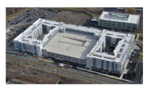
The system provided a maximum allowable footing bearing pressure of 6 kips per square foot (ksf) and was designed to limit total and differential post-construction footing settlement to less than 1-inch and  $\frac{1}{2}$ -inch respectively.
