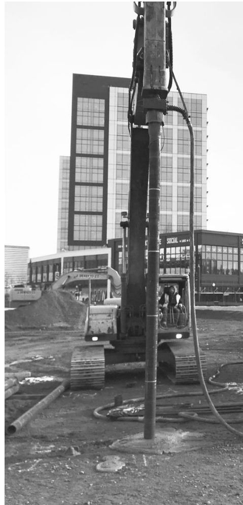
Figure 6: Ductile Iron Pile Installation
